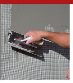
Anti-cracking reinforcement mesh, based on alkaline-resistant fibreglass fibres for better distribution of tension and to prevent cracks from shrinkage, deriving from temperature variations, planar inhomogeneities, etcetera. With a weight of 160 g/m2 and a 4.5 x 4.5 mm square mesh, Armaglass 160 is the ideal fibreglass mesh for creating reinforced skim coats.
