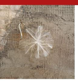
Alkali-resistant fibreglass connector with rigid pre-formed central segment and double-threaded ends. Suitable for the structural reinforcement of brickwork, arches and vaults in masonry, tuff and stone, in combination with ARMAGLASS STRUCTURA fibreglass mesh and mortars such as Unisan, Intosana and the REPAR family. It is used as a conduit for connecting the two sides of structural plaster (with the "structural sandwich" technique).
