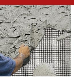
A reinforcement mesh in alkali-resistant fibreglass weighing 225 g/m2, with a 25 x 25 mm square mesh and thermosetting primer equal to about 10% of total weight. Easy and quick to apply, to handle and to cut. It combines lightness and thinness with excellent mechanical characteristics in the warp and weft. Resistant to atmospheric agents and aggressive environments. Suitable for any substrate and perfectly compatible with both cement- and lime-based mortars.
