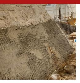
The Armarock B50 basalt mesh is a material with a leno structure, formed by elastic ribs of high-strength basalt threads, fixed in the nodes with a stitching thread, with the formation of square cells, the size of which is ideal for use with FRCM mortars. The mesh is treated with special compounds to improve alkali resistance properties and increase its stability. Balanced biaxial mesh in alkali-resistant basalt fibre, specific for strengthening and repairing structural elements.
