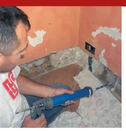
Silane-based impregnating agent with gelatinous consistency for the formation of chemical barriers against capillary rising damp, particularly suited for new masonry, also cellular (refractory bricks, double uni, etc.). It is supplied in 600 cc aluminium-lined bags ("soft" cartridge), to be inserted in the appropriate caulking gun for sealants in bags.
