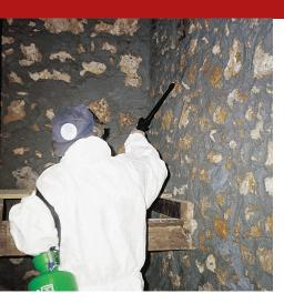
Special balanced solution of fumed silica esters, silanes, siloxanes, in solvent, characterised by high penetrating ability in silicic media and by the effective dual reinforcing and water repellence action, for protective, reinforcing and hydrophobising treatment of mineral and stone media. It does not result in colour variations or alterations of breathability.
