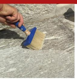
Consilex Idroplus is a concentrated silicone-based product formulated to impart hydrophobic and consolidating characteristics to absorbent mineral building materials, including alkaline materials, natural stones and gypsum. VOC = 0
