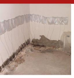
One-component concentrated (60 - 65%) silane-based system modified for the preparation, with the sole addition of water, of water repellent microemulsions for slowly spreading masonry injections against capillary rising damp, specific for the construction of chemical barriers in masonry, brick, tufa, stone and mixed, of varied thicknesses.
