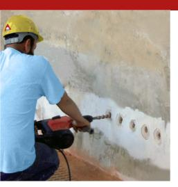
One-component silane-based system modified for the preparation, with the sole addition of water, of water repellent microemulsions for slowly spreading masonry injections against capillary rising damp or using a pump with low operating pressure (0.5 to 1.5 bar), specific for the construction of chemical barriers in masonry, brick, tufa, stone and mixed, of varied thicknesses.
