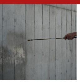
Consilex No-Rust is a powerful non-toxic corrosion inhibitor, to be applied to the surfaces of concrete structures and which, thanks to its particular chemical nature, migrates within the conglomerate and deposits on its particular internal reinforcement substances that preserve their integrity over time, by inhibiting oxidation phenomena.
