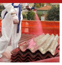
Fixative latex, penetrating, consolidating, flexibilizing reactive type, based on styrene butadiene copolymers in aqueous emulsion, for the temporary encapsulation of type D of asbestos sheets in the uninstallation and removal operations, added with inorganic red pigments, for improve the visualization of the treated surfaces.
