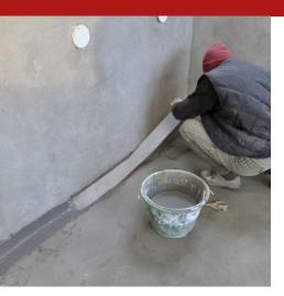
Waterproof butt strap, consisting of a expandable elastomeric rubber, entirely coated on both sides with absorbent fabric, with an overall width of 12 cm. The product is distinctive for its simple and easy application, the ascertained watertightness to water and the high deformation capacity.
