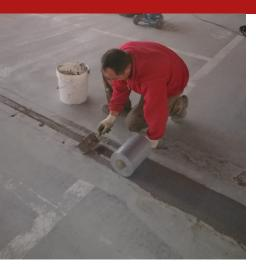
Strap with high resilience and resistance, with an overall width of 25 cm, consisting of a special elastomeric layer in Hypalon, resistant to raging and wear and tear, for use in combination with the epoxy resins paste Syntech AS 21 or Syntech AS 31, for waterproofing watertight expansion joints in buildings, works and structures below the aquifer level or to ensure the water sealing of structural connections even off the ground. Specific applications for industrial or infrastructural use.
