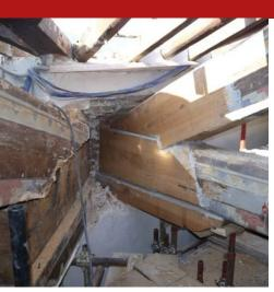
A castable epoxy mortar, comprised of a two-component epoxy adhesive (A + B) to be integrated with a mixture of select mineral aggregates with a maximum diameter of 4 mm. It is used for anchoring, restoring industrial flooring, the localised regeneration of wooden beam heads, repairs and building reconstructions in general, to be completed by pouring on-site, after creating dedicated containment formwork suitably waterproofed with a release agent.
