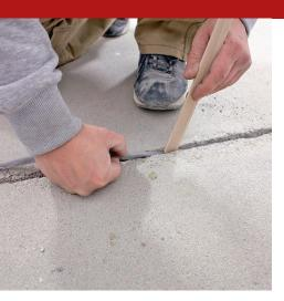
Closed cell polyethylene foam kerb, compressible, to properly size the depth of the expansion joints (creation of the "third wall" or base material) before filling them with the polymeric sealants Protech Flex, PROTECH SIGILFLEX MONO or EG 91. It is available in profiles of circular cross-section of different diameter that will fit joints of any shape and size.
