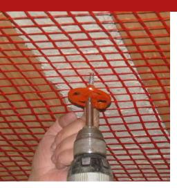
Insulation fastener plastic dowel (58 mm in diameter and 40 mm in length) with screw in corrosion-resistant galvanised steel (30 mm) for connecting ARMAGLASS STRUCTURA mesh in anti-detachment RINFOR SYSTEM 1 and 2.
