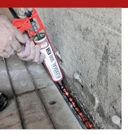
A hydro-expansive polyurethane sealant in a thixotropic paste, pre-packaged in an extrudable cartridge with standard dosing guns, to be utilised as a waterstop in the most complex or problematic situations in waterproofing below-ground areas. Its elastic and sealing properties remain unchanged over time. In a completely dry state, Flexseal 300 shrinks to its original size and then expands again upon contact with water.
