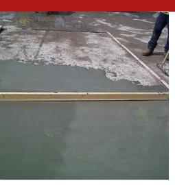
Floor Level SFR is a self-levelling modified-polymer cement mortar having fibre-reinforcement with Readymesh MR-060, offering accelerated grip and fast hardening. Applied prior to laying the flooring, it is perfect for levelling at thicknesses ranging from 3 mm to 25 mm so as to adapt to any type of covering.
