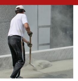
A premixed hardening mineral blend with a base of basalt, corundum, high-purity quartz, super-pozzolanic reactives (thickened microsilicates) and hydraulic binders for surface armour dust or paste, for industrial concrete flooring.
