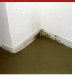
Floorband 200 – comprised of closed-cell polyethylene and being lightweight, waterproof, imputrescible, mould-proof and with a high resistance to chemical aggression and alkaline reactions of cementitious products – is mainly used as a perimeter insulating band during the construction of screeds and/or concrete flooring.
