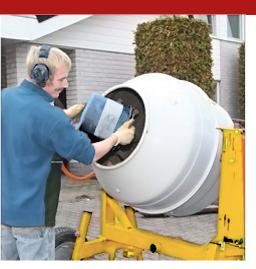
Fluid Hydro is a special aqueous emulsion additivated with white water-repellent products consisting of active components with an alkyl-silane base. The main characteristic is the property of reducing water permeability in concretes, plasters and mortars both due to the capillarity and lashings of water.
