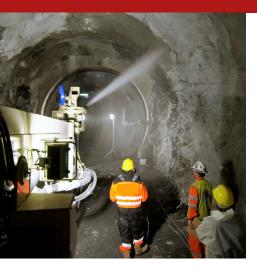
Solution of mineral reactives (sodium silicate) to be used for the acceleration of setting of sprayed masonry and projected concretes, in the reinforcement of rocks outdoors and/or in a gallery, in laying self-sustaining and waterproofing claddings of tunnels, channels, vaults, basins, underground structures, etc., for use with specific equipment for hydrated mixtures (mixtures in which the silicate is sprayed on the shotcrete output nozzle).
