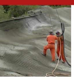
Alkali-free mineral reactivity solution to be used to accelerate sprayed concrete and shotcrete, in the consolidation of rocks outdoors and/or in tunnels, in the construction of self-sustaining and waterproofing coatings of tunnels, canals, vaults, basins, underground works, etc., to be used both dry and wet directly in the mix design of the concrete to be sprayed.
