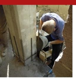
Grout 2 SFR is a high-performance, self-levelling castable mortar, being fibre-reinforced with Readymesh MM-150 steel fibres and Readymesh PM-060 polypropylene microfibres, with high flexural strength, great adhesion to concrete and steel, and shrinkage compensation. Aggregates with a maximum size of 2 mm. It is ideal for restorations, reinforcements and seismic adjustments, offering ductility for medium thicknesses (3-10 cm), on structures in reinforced concrete and masonry.
