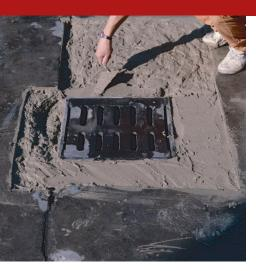
Castable mortar, reinforced with steel fibres, fast-curing, based on portland cement, special binders, selected siliceous aggregates and specific rheologic agents, for repairs, reconstructions and anchorages for fast re-use, in road works and in concrete, even in severe weather conditions and at low temperatures.
