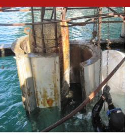
Composite, castable, anti-washout, controlled shrinkage cement mortar, superfluid consistency, based on high-resistance cements, superpozzolanic fillers (MICROSIL 90), polymeric modifiers, shrinkage resistant agents, specific additives, calcium silicate mineral fibres, selected silica aggregates.
