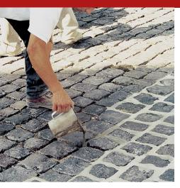
An anti-shrinkage, pourable, self-levelling, super-adhesive micro-mortar, based on high-strength cements, super-pozzolanic fillers, polymeric stabilisers and anti-shrinkage agents. Aggregates with a maximum size of 0.35 mm. Ideal for filling joints (gaps and/or interstices) in urban paving made of porphyry or stone slabs, even of large dimensions. For filling cracks and lesions on concrete and masonry structures.
