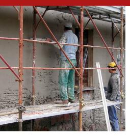
Premixed, fibre-reinforced, breathable plaster, based on hydraulic lime, for coating and repairing internal and external walls and masonry, for new buildings, existing buildings, ecological building interventions, in new buildings and in the restoration of vintage buildings and monuments.
