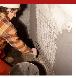
Osmotic fibre reinforced two-component cement mortar, based on hydraulic binders, modifying resins and flexibilisers, superpozzolanic reactive fillers, for the preparation of adhesive mixtures, easy to spread, which after hardening, provide an effective waterproofing protection, both in direct push and in negative pressure, with high capacity of deformation.
