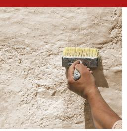
Osmotic brushable hydraulic lime-based compound, for the construction of vertical barriers, waterproofing, in porous structure masonry (brick, natural stone, etc.) in ecological building interventions, new buildings and in the restoration of vintage buildings and monuments.
