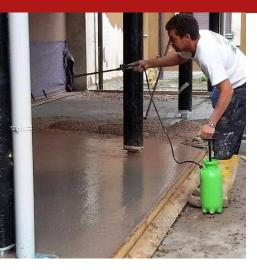
Set retarder in aqueous solution to be applied, using a low pressure airless pump, on fresh concrete surfaces, to allow removal by washing with water, a cortical layer a few millimetres thick, and then expose the aggregate forming the concrete. Specific for the realisation of floors with landscape/environmental value with the "washed gravel" technique.
