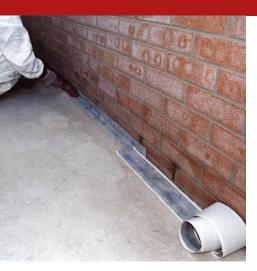
Cold applied water-repellent adhesive tape, composed of a layer with visco-elastic butyl rubber consistency, coated with a polypropylene non-woven fabric, for elastic waterproofing of non-structural joints in balconies, terraces, etc. Size of the strap: 80 mm x 0.9 mm.
