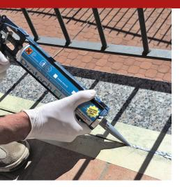
A single-component, moisture-curing and fast-hardening polyurethane sealant with a medium-to-high modulus of elasticity, remaining permanently elastic yet with high surface hardness and being tear- and weather-resistance and paintable. Ideal for the deformable sealing of expansion joints on terraces and balconies, for filling joints on prefabricated walls and on wooden, steel, aluminium, copper and plastic materials along with plasters and so on.
