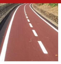
Protech Road Paint is a thick paint based on acrylic resins in aqueous emulsion for the protection and waterproofing of bituminous floors in urban and pedestrian areas. Protech Road Paint is ideal for surfaces in car parks, yards, cycle paths and sidewalks, it also increases the resistance of the floor to wear, UV rays and chemical aggression.
