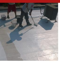
Protective and waterproofing liquid coating, single-component, coloured, based on special elastomeric polymers in aqueous emulsion, suitable for the waterproof protection of flat roofs, pitched roofs, attics, walkable terraces, old bituminous coverings and external areas subject to atmospheric agents. The product is resistant to UV rays and water stagnation. It can be advantageously used as an elastomeric paint for the protection of concrete infrastructures and cementitious supports in general.
