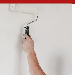
Anti-condensation, elastic, sanitizing, heat-reflecting paint, with hollow glass microspheres (3M Glass Bubble), ideal for both external and internal facades, based on siloxane resin in emulsion, with high permeability to water vapor and with excellent covering power. Recommended as a breathable, water-repellent protective finish for macroporous dehumidifying plasters (Sanatigh, Sanawarme, Caleosana).
