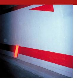
Tempera paint with high specific coverage, high dry residue and discrete water repellence, for painting signs and decorative interior surfaces generally relating to tunnels, galleries, subways, etc. Pure white: RAL 9010 Vermilion: RAL 2002
