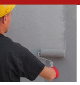
Single-component colored finish in water dispersion for the opaque protection of concrete surfaces and cementitious substrates, wall coverings, and appropriately prepared and primed floors. The product is a painting system suitable for environments with the presence of food, which can be used to protect walls and ceilings that comply with the HACCP protocol, in order to prevent possible food contamination.
