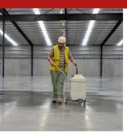
A sodic impregnating agent of polysilicic acid in aqueous solution (sodium silicate) for antidust and protective treatments of concrete flooring and screeds. It drastically reduces the product's water permeability whilst maintaining the passage of aqueous vapour. Consequently, the resistance to acid attacks and the overall durability of the concrete work increases.
