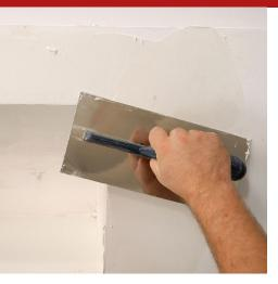
Structural, fibre-reinforced thixotropic cement skim coat, with excellent adhesion characteristics, resists compression, bending and abrasion, etc. Ideal for structural renovation of works and manufactured pieces in deteriorated concrete. Apply using a trowel.
