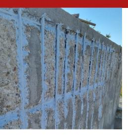
Cement slurry in monocomponent powder, passivating, light blue in colour, to be added with water, modified with superpozzolanic agents, flexibilising resins and corrosion inhibitors, for the passivating treatment of oxidised reinforcing rods, in the restoration of degraded concrete.
