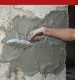
A single-component, super-adhesive cementitious mortar for rough coating, with a base of high-strength binders, selected aggregates, adhesion-promoting polymers and specific agents. Ideal for the preliminary "rough coat" treatment of concrete surfaces, mixed masonry, rock walls and other poorly-absorbent surfaces, for subsequent coating with traditional (Intosana), dehumidifying (Sanatigh) and/or thermal-insulating (Sanawarme or Caleosana) plasters.
