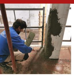
Structural, thixotropic, rheoplastic, composite cement mortar, based on high-resistance cements, superpozzolanic fillers, polymeric modifiers, anti-shrink agents, plasticisers, stabilisers, anti-corrosive, anti-allergic additives, selected aggregates, polypropylene fibres.
