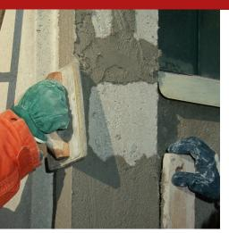
Structural cementitious mortar, two-component, composite, with compensated shrinkage, fiber-reinforced, based on high-strength cements, super-pozzolanic fillers, water-dispersed polymeric resins, migratory corrosion inhibitors, anti-shrinkage additives, plasticizers, stabilizers and anticorrosion agents, selected aggregates, READYMESH microfibers in glass, with a high zirconium content, and multifilament polypropylene.
