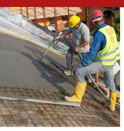
High-performance, thixotropic, structural cementitious mortar, fiber-reinforced with a mix of metal microfibers (length = 6 mm, diameter = 0.22 mm) and alkaline-resistant synthetic microfibers, used for the restoration and thickening of reinforced concrete structures and in masonry, even in severe exposure environments (marine, industrial, cyclically dry and wet).
