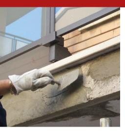
Structural, rheoplastic, thixotropic cement mix with controlled shrinkage, with adequate super-pozzolanic filler additives, hold accelerators and glass micro-fibres. The mix is equipped with very fast hold, excellent workability and excellent adhesion on cement supports to rebuild. The product was mainly designed for small/medium repairs and reconstructions in environments where the fastness of application is important, such as works on roads, ports and airports.
