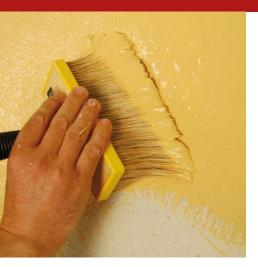
Breathable, natural, non-toxic paint, for internal and external surfaces, diffusive type, based on lime putty. Mineral-based, active formulation, high natural anti-mildew and anti-condensation capacity, prepared according to the traditional recipes, for use in ecological building interventions and in the restoration of vintage buildings and monuments.
