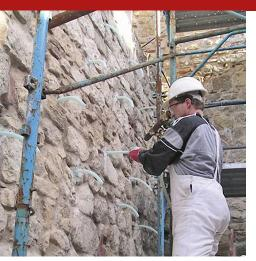
Powder preparation, ready-to-use, based on hydraulic lime, for the preparation, with the sole addition of water, of grout for masonry reinforcement, injectable and castable, high performance in terms of sliding, strength and stability, for ecological building interventions and the restoration of vintage buildings and monuments.
