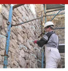
Powder preparation, ready-to-use, based on hydraulic lime, for the preparation, with the sole addition of water, of grout for masonry reinforcement, injectable and castable, high performance in terms of sliding, strength and stability, for ecological building interventions and the restoration of vintage buildings and monuments.
