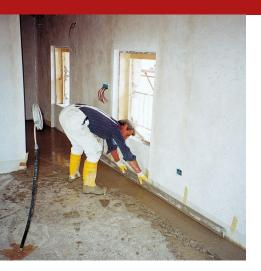
Walkable screed based on hydraulic lime, silico-calcareous aggregates with a maximum grain size of 5 mm and light aggregates with pozzolanic activity, fiber-reinforced with polypropylene and glass microfibres, used for the construction, with the addition of water, of resistant screeds and substrates , in green building interventions and in the restoration of period and monumental buildings.
