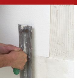
Flexible membrane with thermal insulation and vapor barrier properties, made on a nonwoven fabric support made of 100% recycled polyester, coated with a specific flameretardant acrylic compound, 100% water-based.
